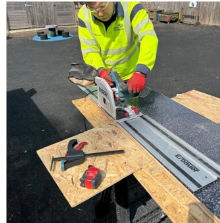
A colleague spent two days renovating a nursery
