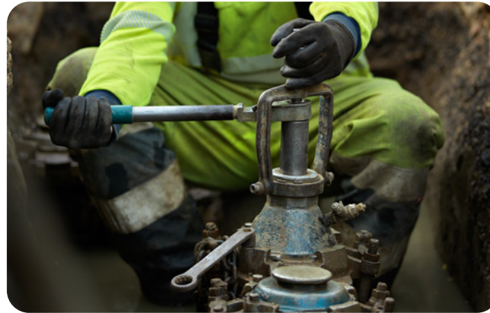
Gas mains replacement work
