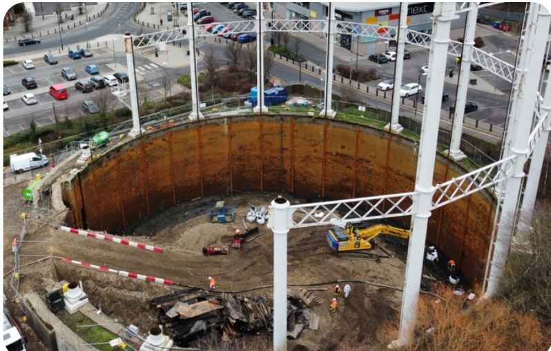
South Shields gas holder demolition, image courtesy of Erith Ltd
